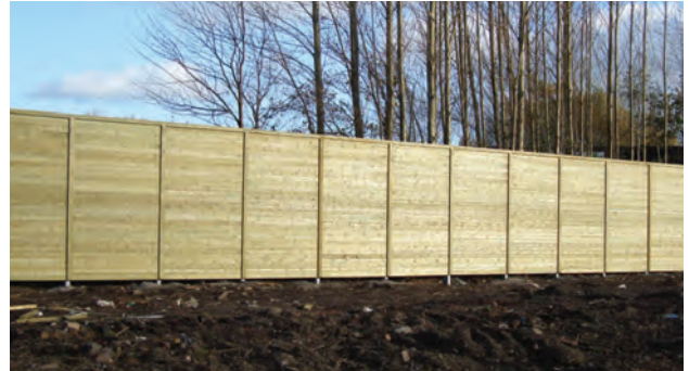
Torwood - 450m of Jakoustic Highway from 4m to 6.5m high
